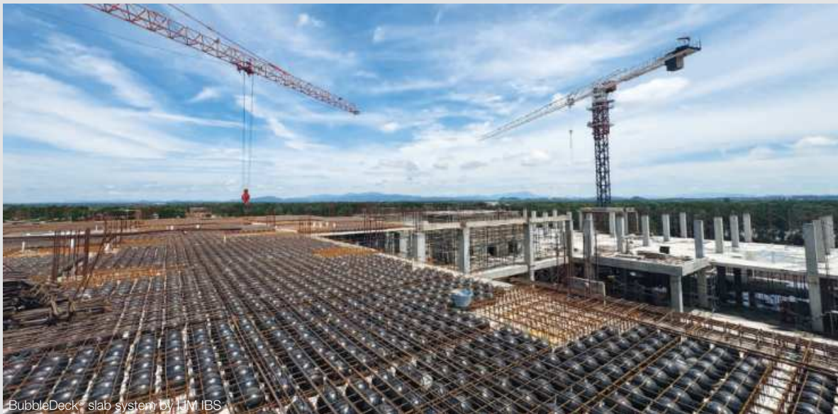
BubbleDeck® slab system by IJM IBS
