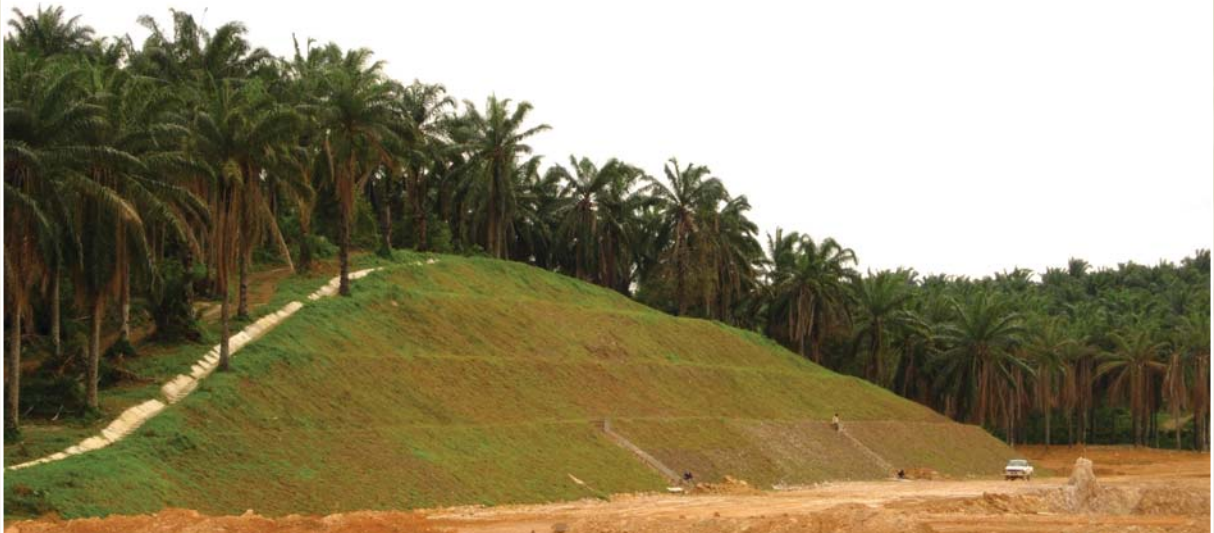
Turfing to prevent slope failure
