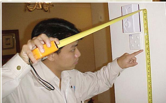
Checking of electrical switch position
