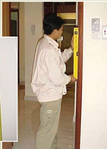
Checking of door frame alignment
