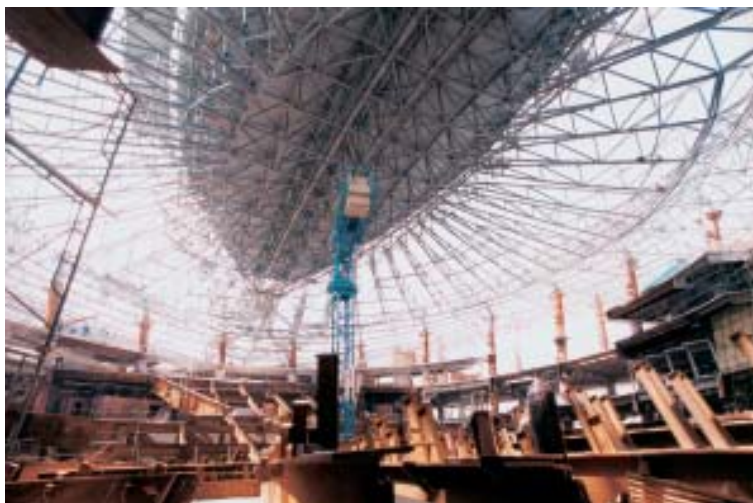
Main roof steel structures fabricated by Torsco for Putrajaya Convention Centre
