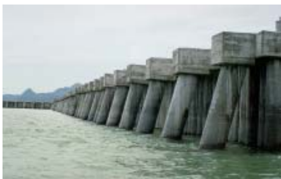
Breakwater at Royal Langkawi Yacht Club using ICP Piles
