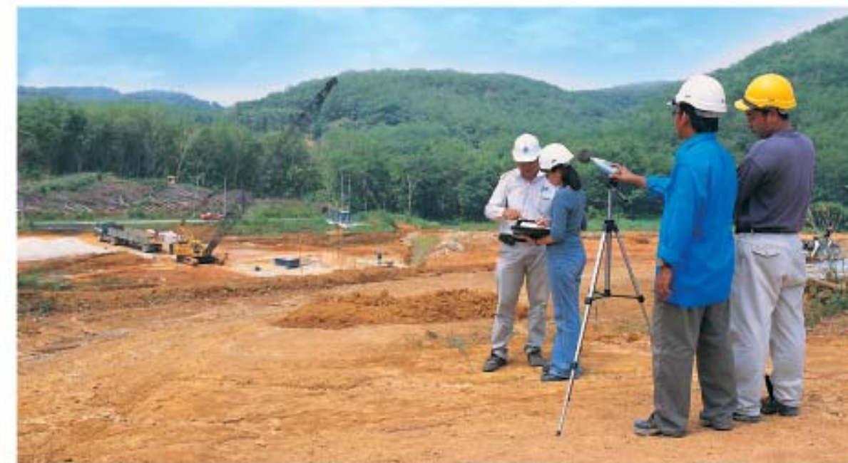
Measurement of noise level generated by construction machineries at an open space within the nearest residential area of Jalan Lingkar Bandar U4 project in Putrajaya
