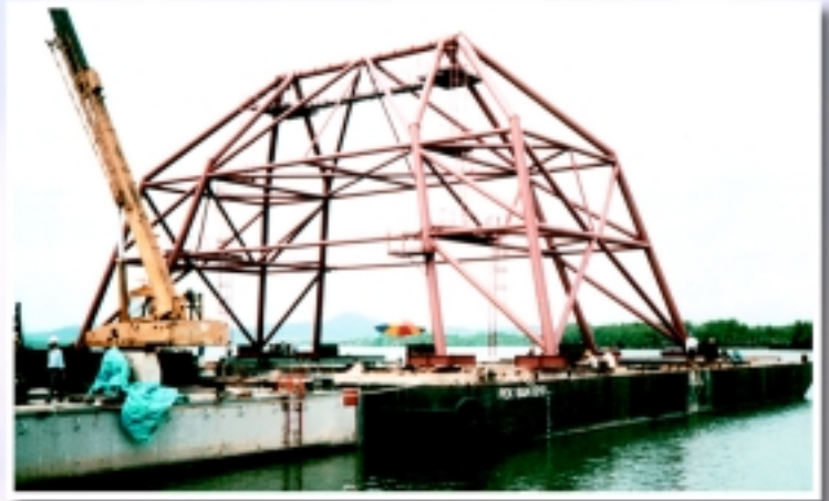
Load-out of Kangaroo Crane onto two barges at Plant No.3, Lumut for TNB Janamanjung project
