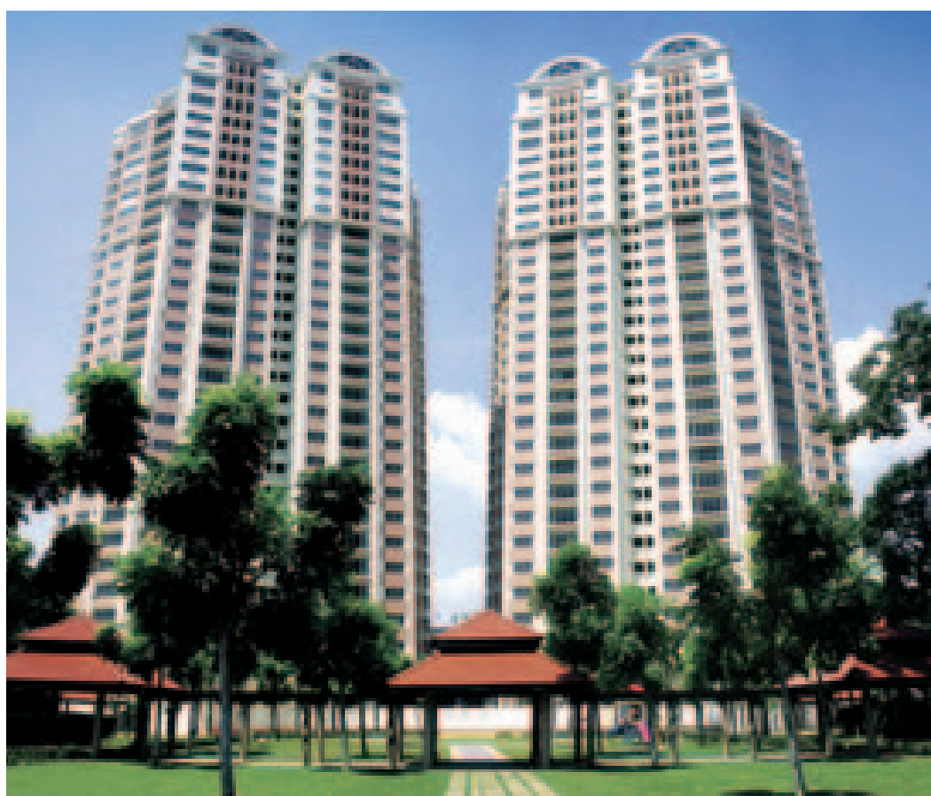
Kondominium Boulevard, Subang Jaya
