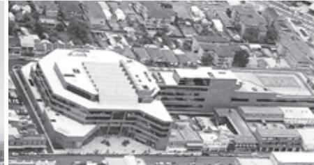
Bangunan St George Building Society, Sydney, Australia
