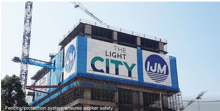
Fencing protection system ensures worker safety
