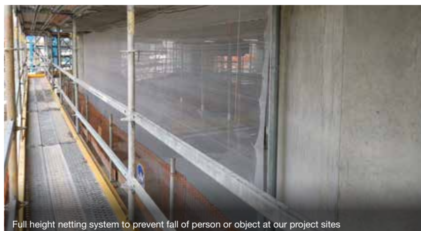
Full height netting system to prevent fall of person or object at our project sites
