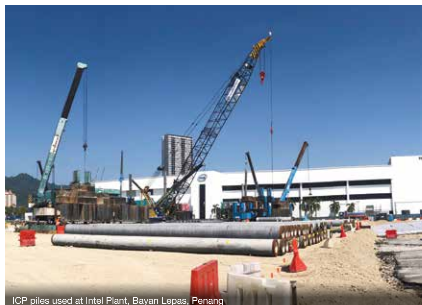
ICP piles used at Intel Plant, Bayan Lepas, Penang
