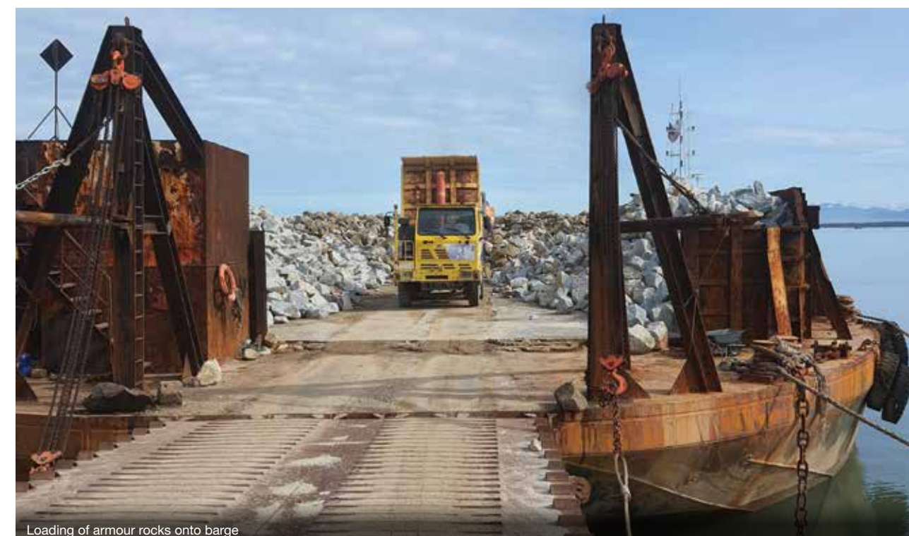
Loading of armour rocks onto barge
