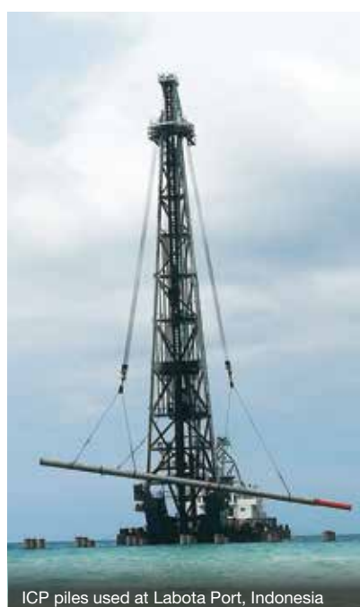
ICP piles used at Labota Port, Indonesia
