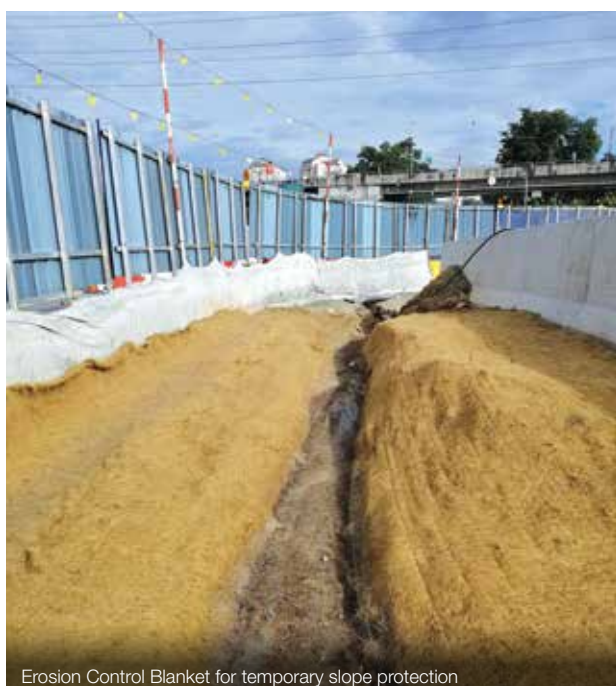
Erosion Control Blanket for temporary slope protection
