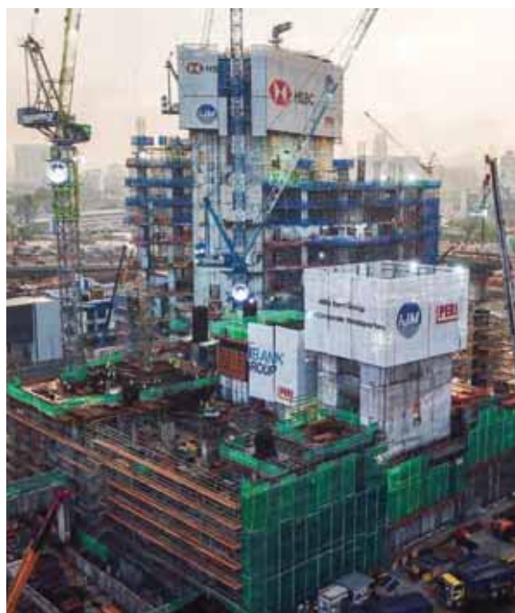
Screen system offers added safety and protection in the construction of high-rise buildings
