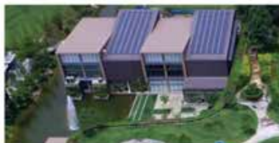
PV solar panels installed on the sales gallery building roof
