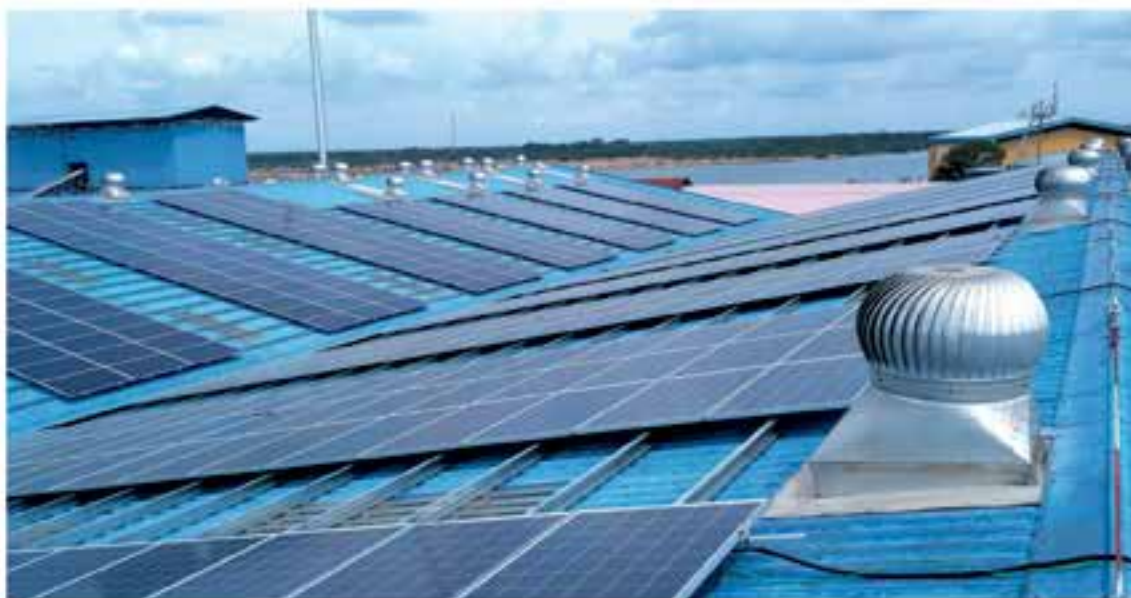
Rooftop solar PV system at Lumut factory
