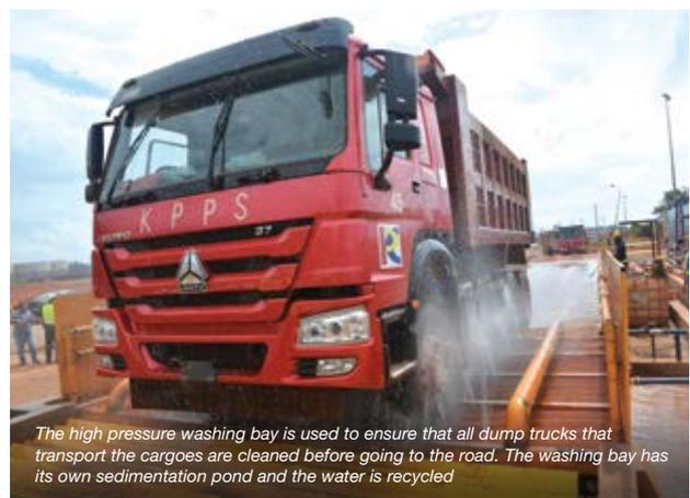
The high pressure washing bay is used to ensure that all dump trucks that transport the cargoes are cleaned before going to the road. The washing bay has its own sedimentation pond and the water is recycled
