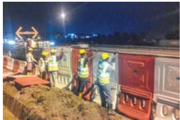
Installation of hoardings to contain dust and noise pollution
