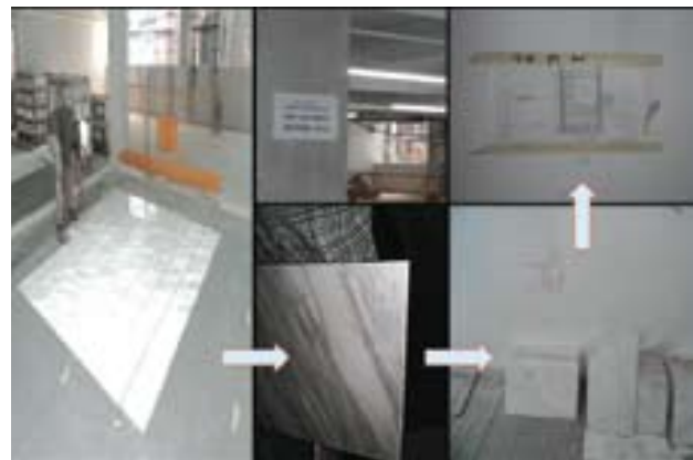
Marble tiles are dry laid in accordance with its design and tonality
