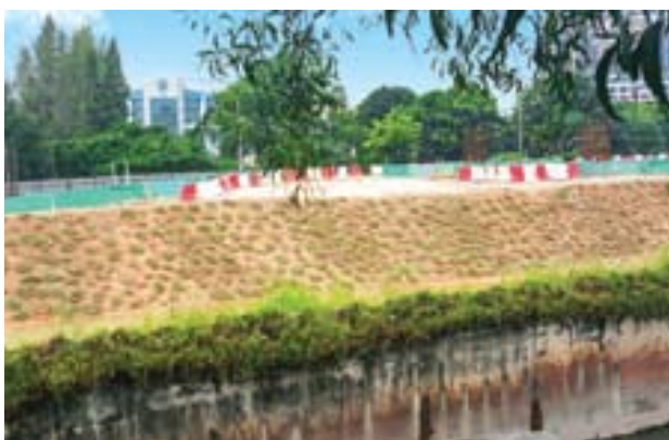
Spot turfing as slope protection
