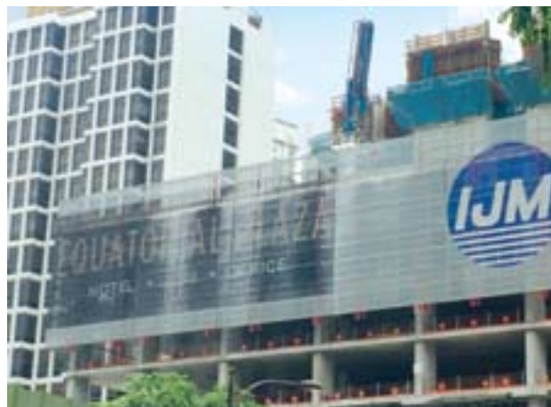
Installation of screen system at construction site
