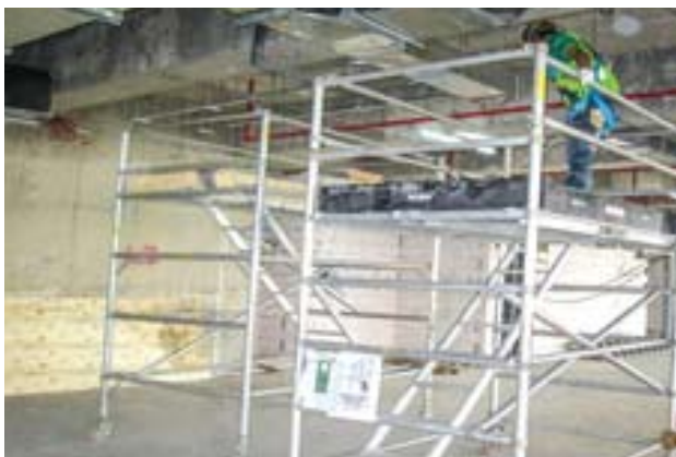
Working platform erected for workers at site
