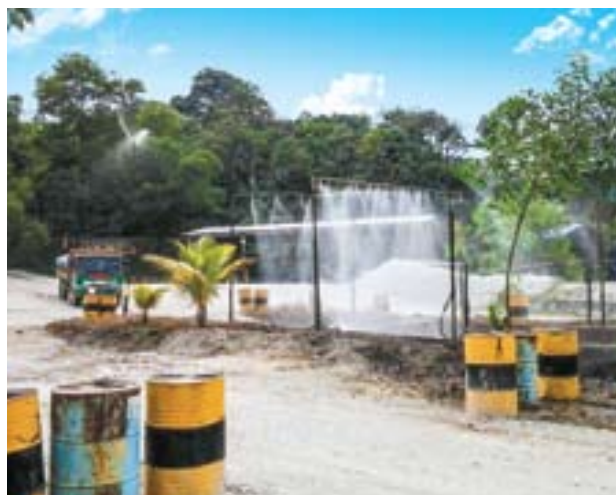
Washing bay is important to wet the dry particles to avoid it being blown away
