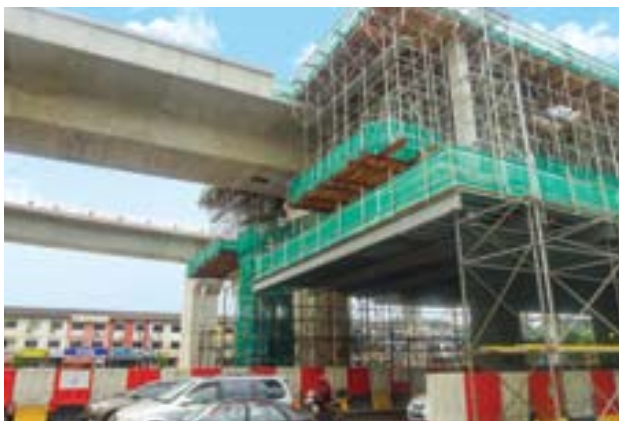
Installation of overhead protection while working above live traffic
