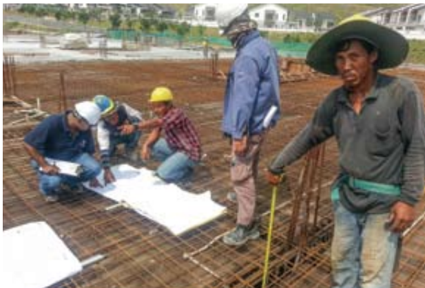
Structural IQSAS assessment on reinforcement as pre-concreting works is in progress at Phase 2R, Seremban 2 Development Project
