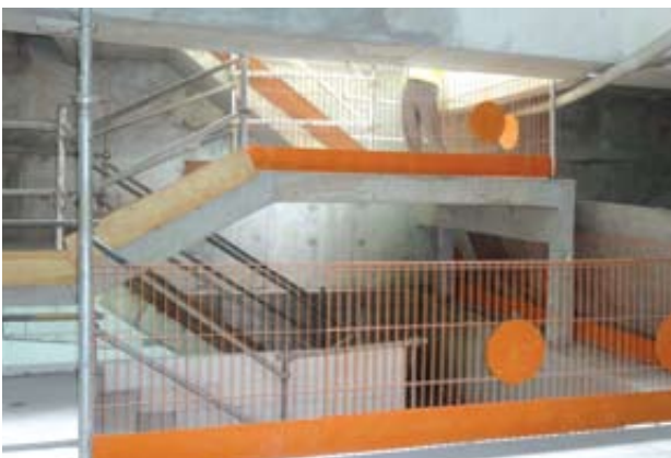
Installation of fencing to prevent falling hazard
