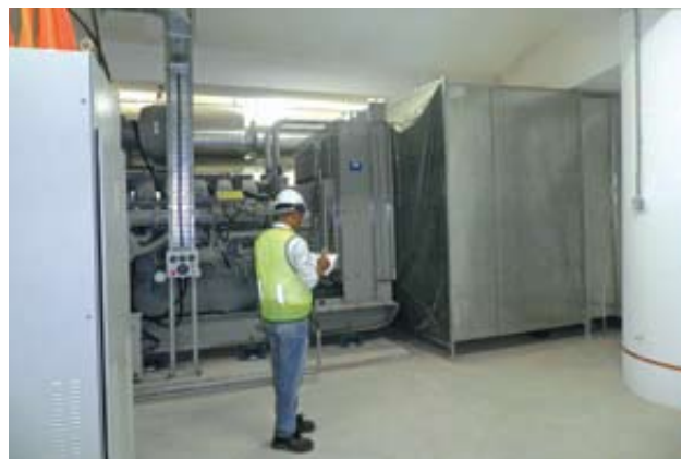
Inspection and assessment of Air Conditioning Mechanical Ventilation Equipment
