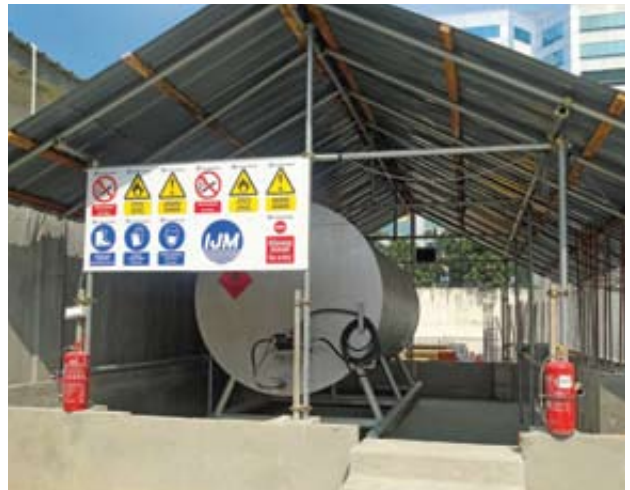
On site diesel storage equipped with safety signage, fire extinguisher and concrete bund
