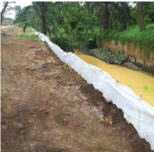
Silt fencing along the drain and river as an erosion and sedimentation control measure
