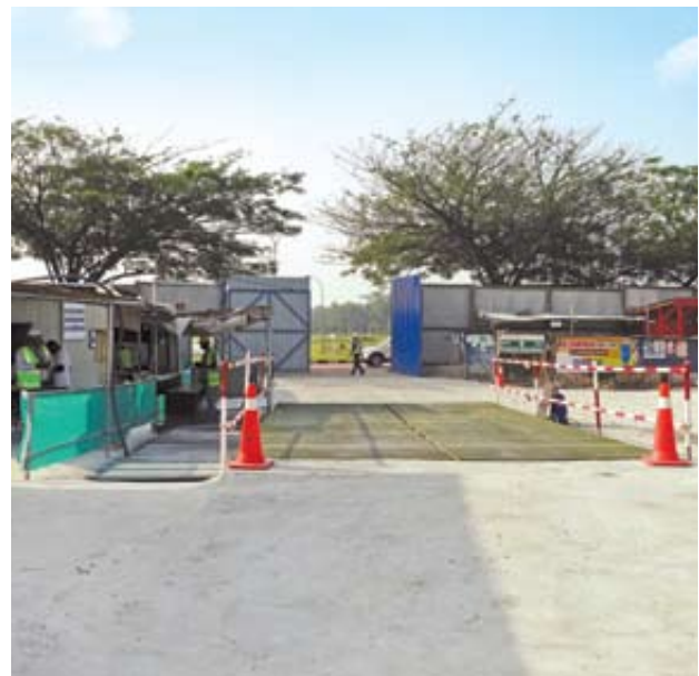
Wheel washing facility at site entrance to contain dust pollution
