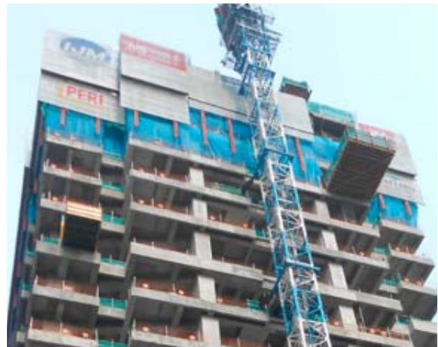
Screen system is installed at construction site
