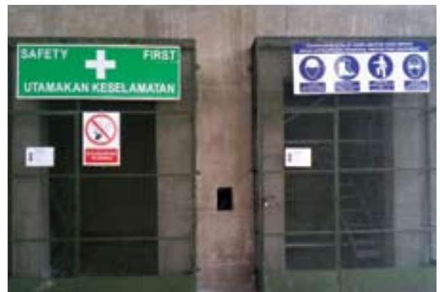
Entrance to lift shafts protected with full height tamper-proof locked gates with warning signs displayed
