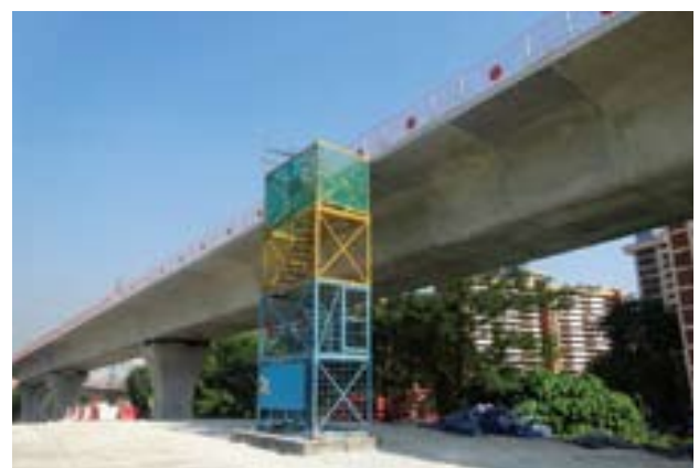
Installation of fencing system for prevention of falling hazard
