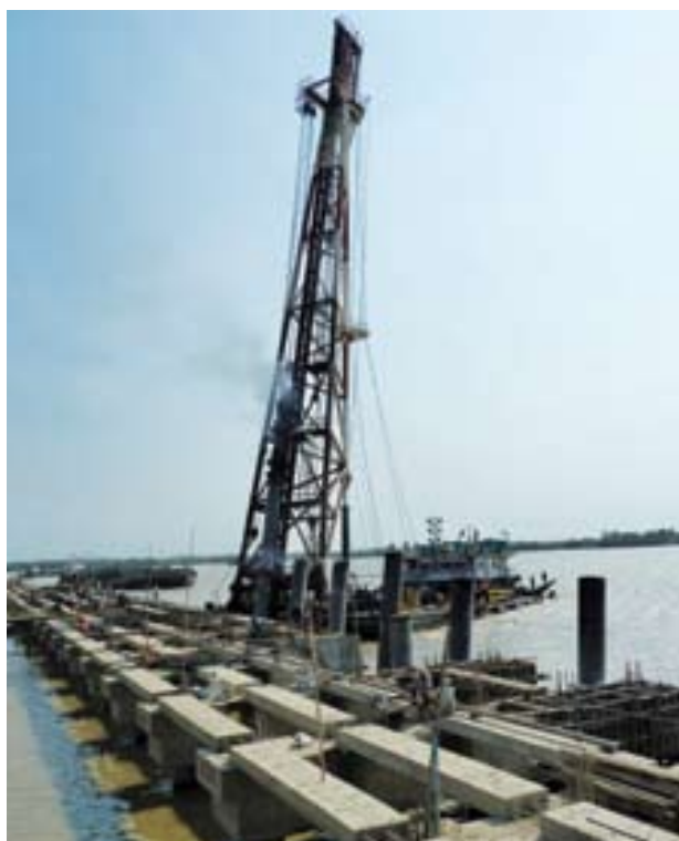
ICP Piles used at Ahlone Container Terminal, Yangon, Myanmar
