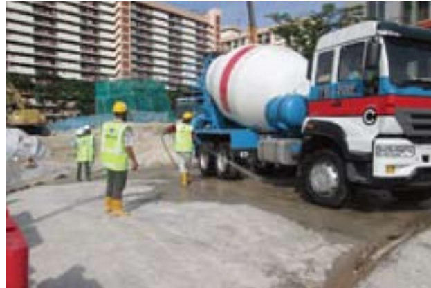
Wheel washing facility to control dust dispersion and ensure public road cleanliness
