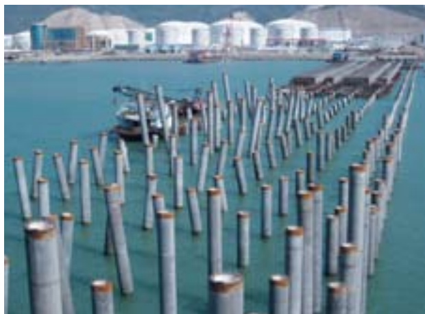
ICP Piles used at Baota Petrochemical Terminal at Zhuhai, China
