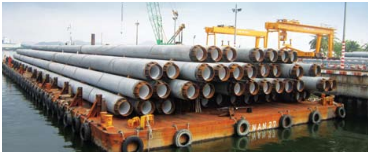
Loading of ICP Piles for shipment at ICP Lumut Jetty
