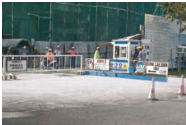
Safe entrance with separate access for workers and construction vehicles
