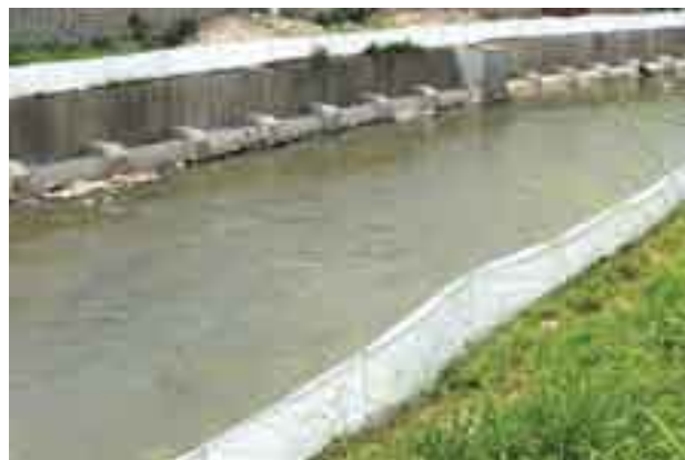
Provision of silt trap for erosion and sediment control at construction site
