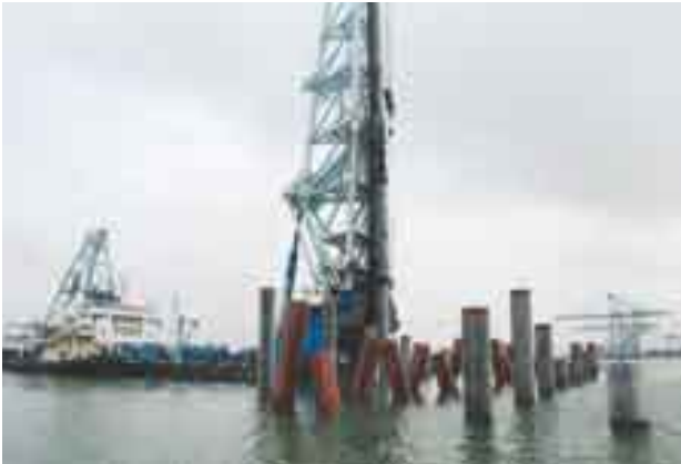
ICP Piles used at the Zhuhai Port International Container Terminal, Zhuhai, China
