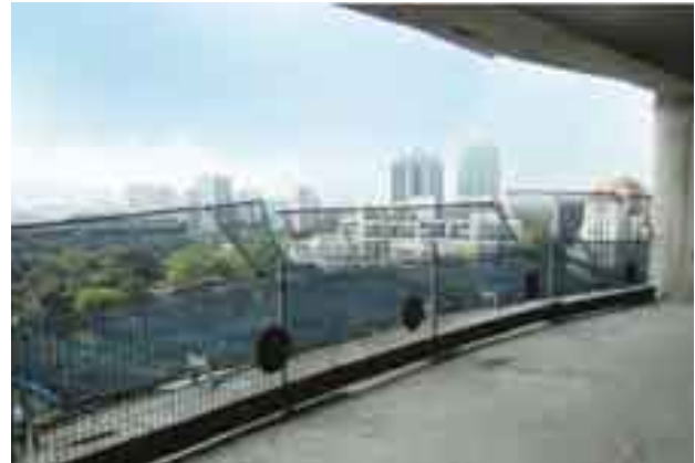
Fall Arrest Safety Nets prevent falling debris from causing injury to people underneath
