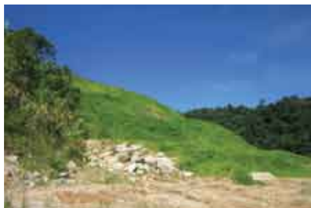
Erosion control mechanism - Hydroseeding
