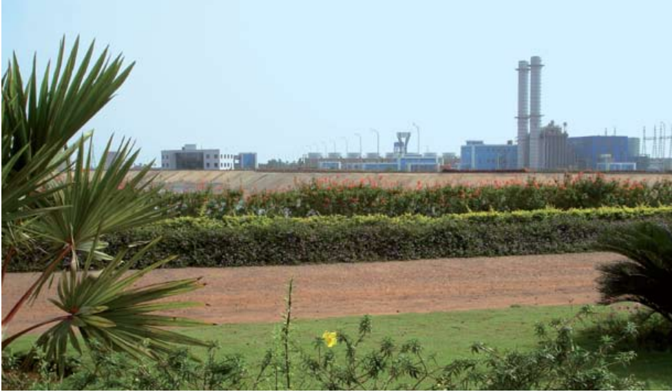
Gautami Power Plant, Andhra Pradesh, India
