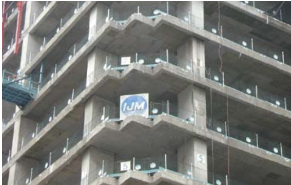
Edge Protection Fencing System prevents falling from high rise buildings under construction
