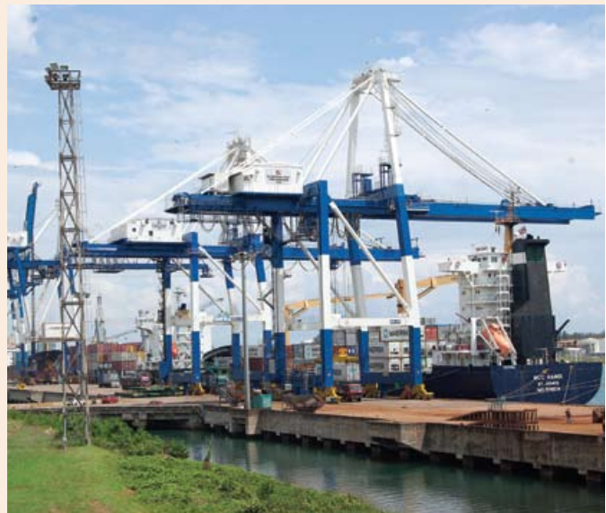
Unloading operations at Kuantan Port, Pahang
