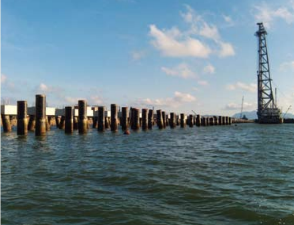
ICP Piles used at Shenhua Coal Terminal Port, Zhuhai, China
