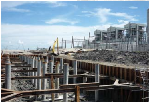
ICP Piles used at Jana Manjung Power Station, Manjung, Perak
