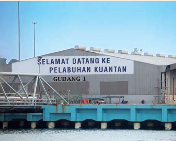
Wharf front warehouse at Berth No.1, Kuantan Port
