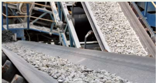
INDUSTRY Conveyor System, Labu Quarry, Negeri Sembilan
