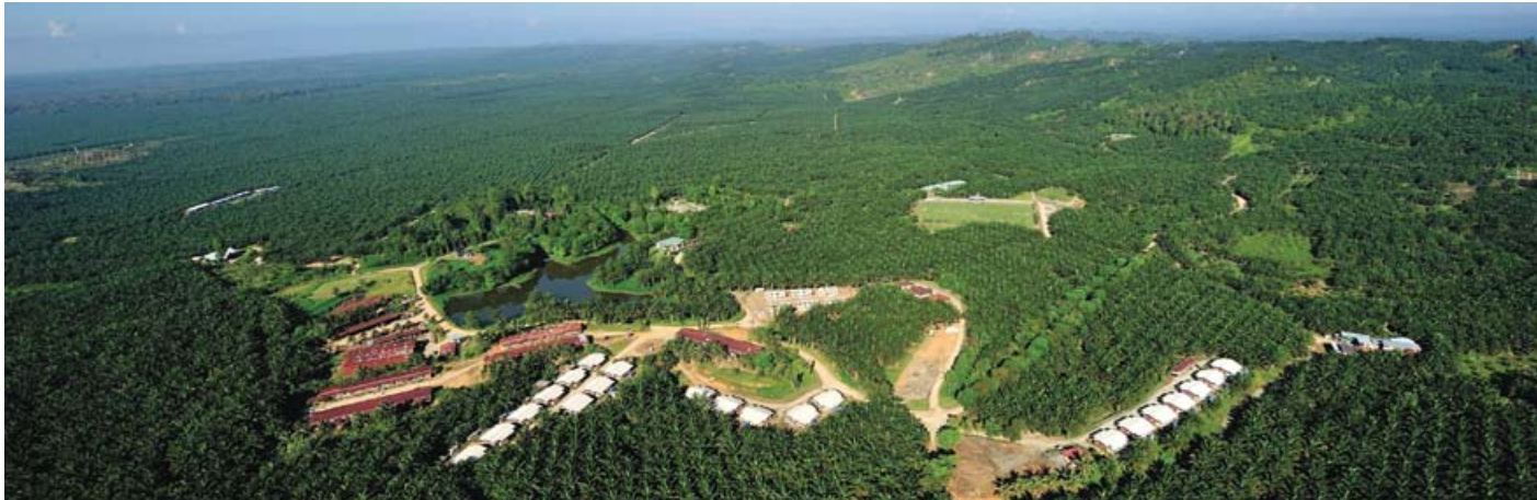
Aerial view of Sungai Sabang Estate
