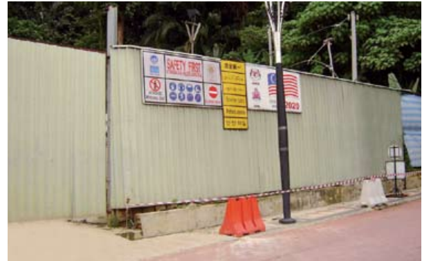
Installation of hoardings to reduce noise pollution
