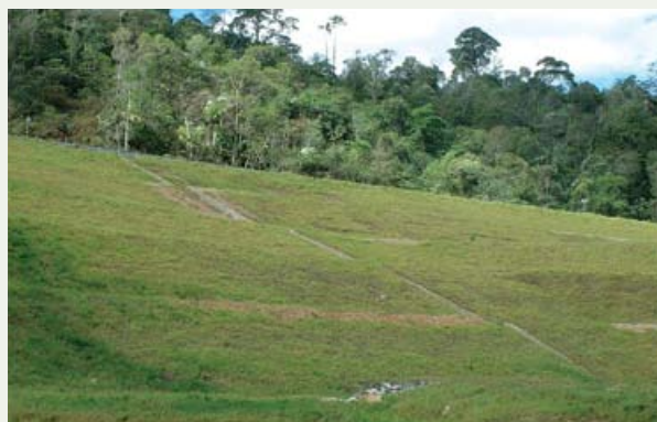
Turfing of slopes to prevent soil erosion
