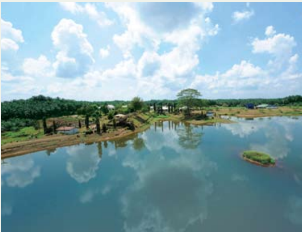
Water catchment at Minat Teguh Estate
