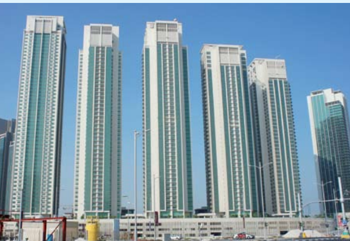
Al Reem Island mixed development project in the Middle East
