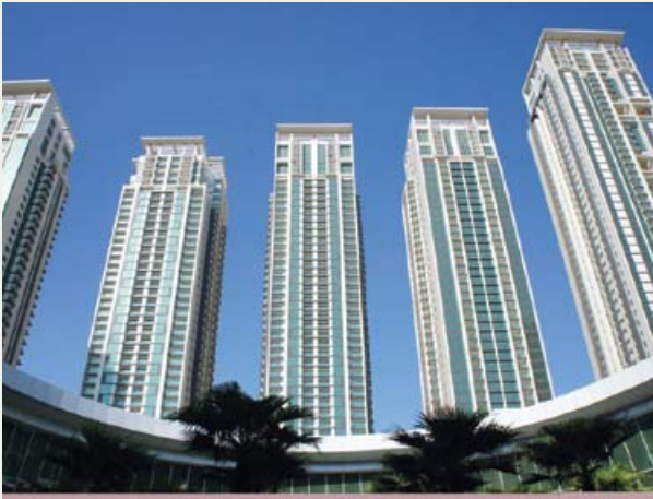
Al Reem Island mixed development project in the Middle East
