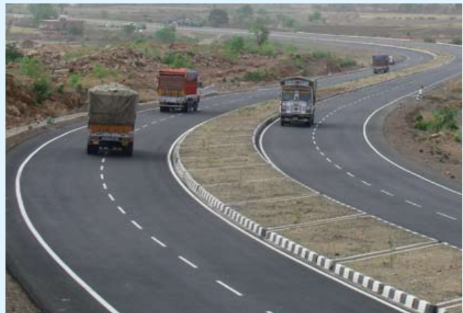
Rehabilitation & Upgrading of Jhansi-Lakhandan road, Madhya Pradesh, India
