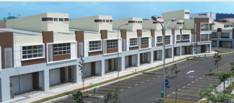
CONSTRUCTION Bukit Raja Shop Office Phase 2, Shah Alam
