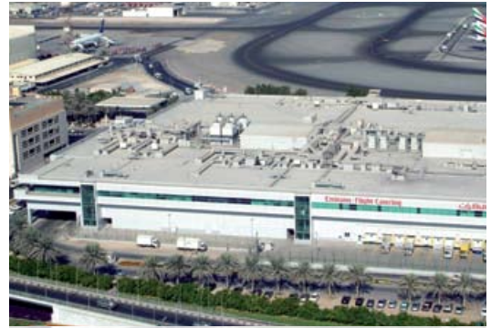
Emirates Catering Facility, Dubai
