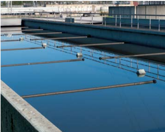
Binh An Water Treatment Plant, Vietnam
