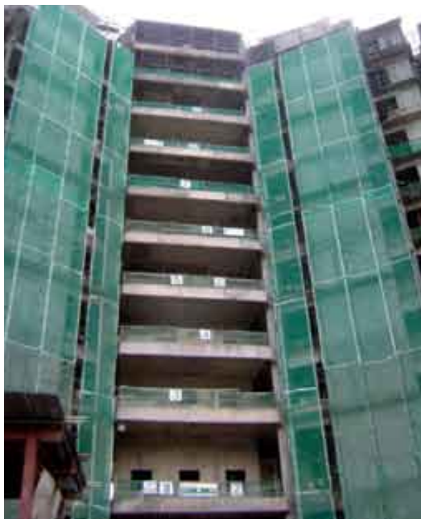
Edge Protection Fencing System prevents fall from high rise building under construction
