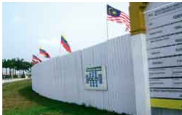
Construction site hoardings used to reduce noise and dust pollution
