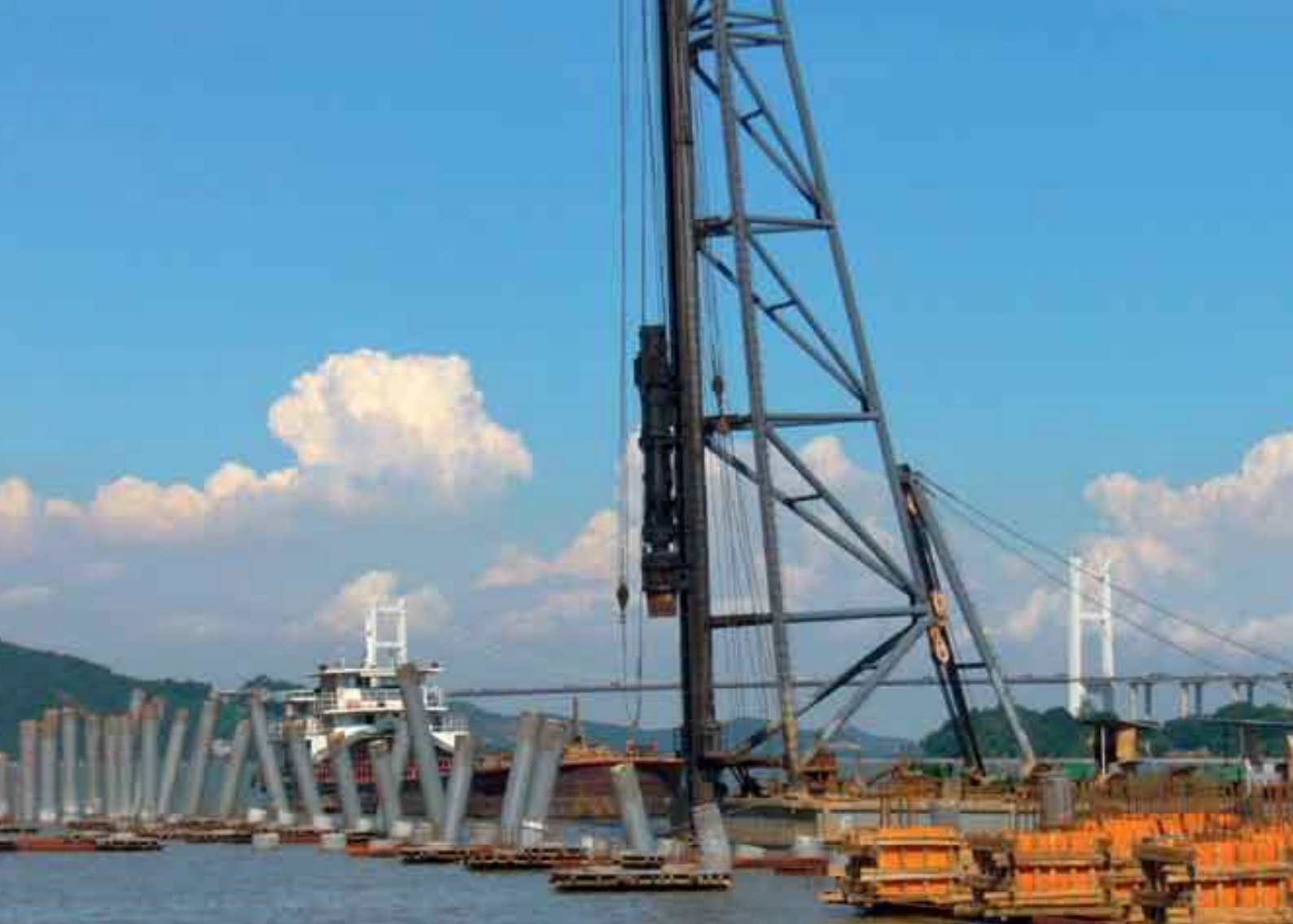
ICP Piles used at the Nansha Maritime Safety Department Jetty, China
