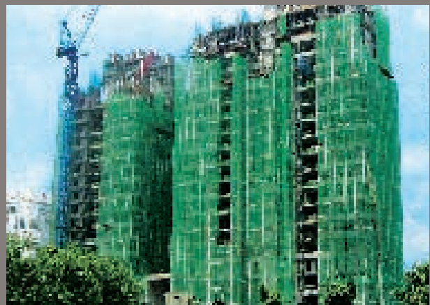
Peripheral netting is practised at building sites for safety
