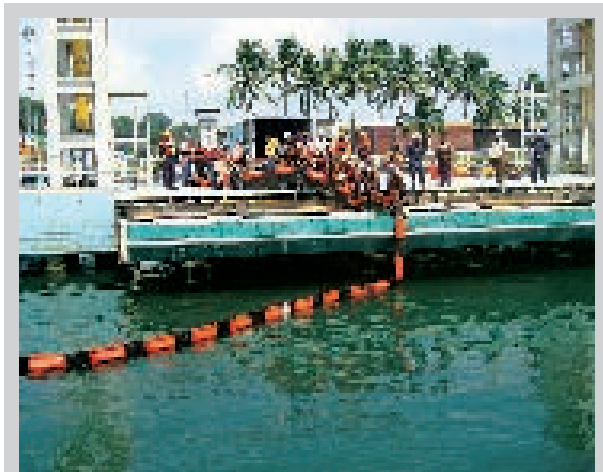
Oil spill exercise where an oil boom is released into the Kuantan Port water basin to restrict the spread of leaked oil
