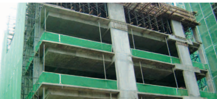
Safety: Edge protection and peripheral netting are practised at our project sites
