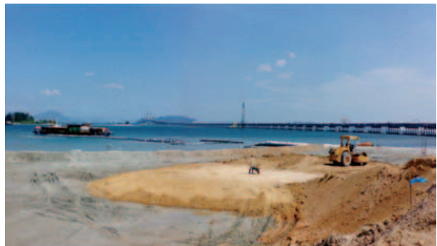
Sand bunds are constructed along the filling perimeter to prevent sea pollution during land reclamation
