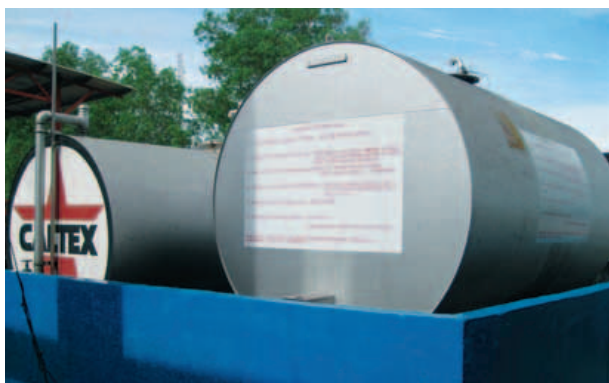
Skid tanks are enclosed by perimeter concrete wall to prevent oil spillage at the factories and surrounding areas under the requirement of OSHA 1994
