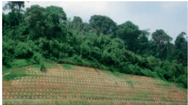
Soil nailing is used to stabilise the earth and prevent landslides at our project sites
