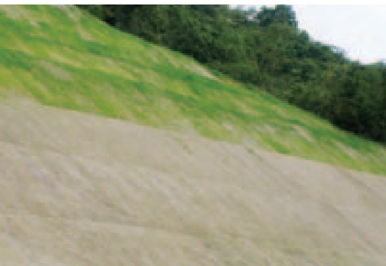
Hill slopes turfing and hydro-seeding are implemented at work sites to prevent soil erosion and land slides
