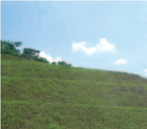
Vegetative cover to protect slope at the Lekas project site
