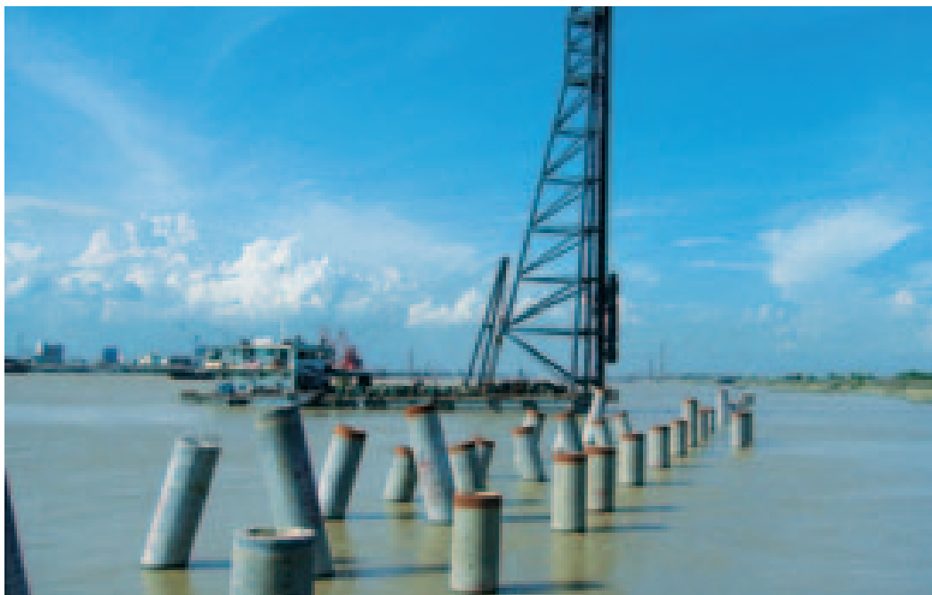
ICP piles used at the Haiwan Petrochemical Port, Dongguan, China
