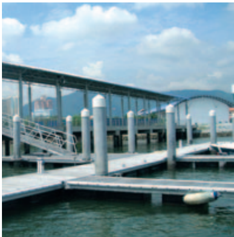
ICP piles used at Marine Police Jetty, Penang
