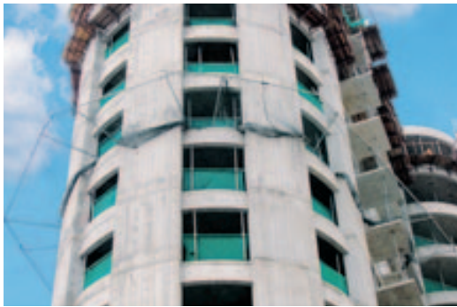
Use of scaffolding and safety net at the Group's PJ8 development
