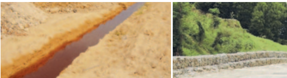
Silt trap and slope stabilisation are some of the environmental measures adopted at our construction sites
