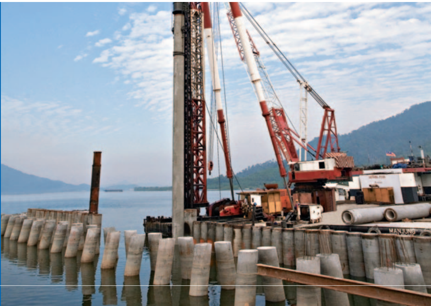
Installation of ICP piles for a marine project
