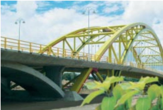
The 130m span steel arch bridge, Batang Mukah, Sarawak
