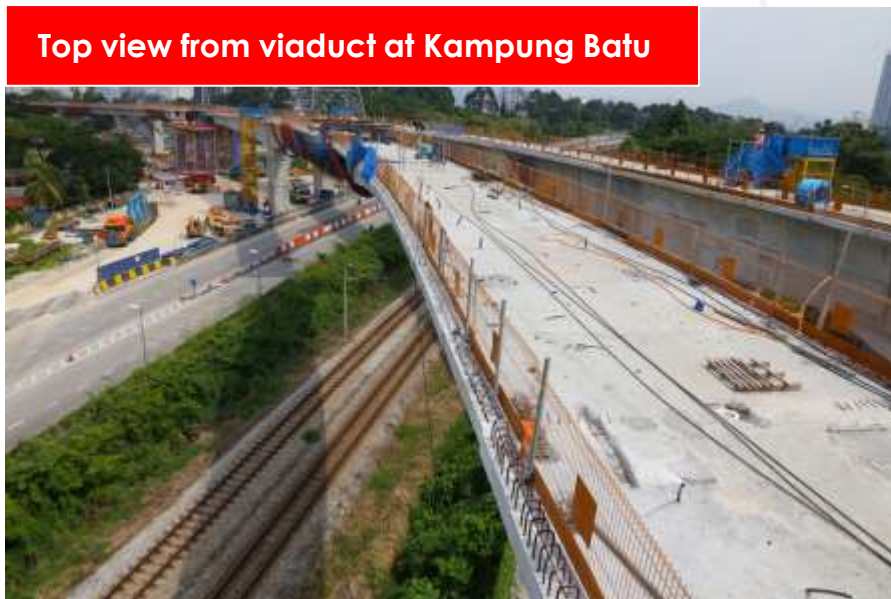
Long span launching at Kampung Batu
