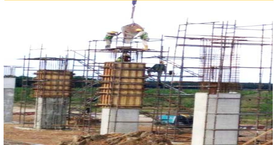
Concrete Casting Work for Bridge Plinth
