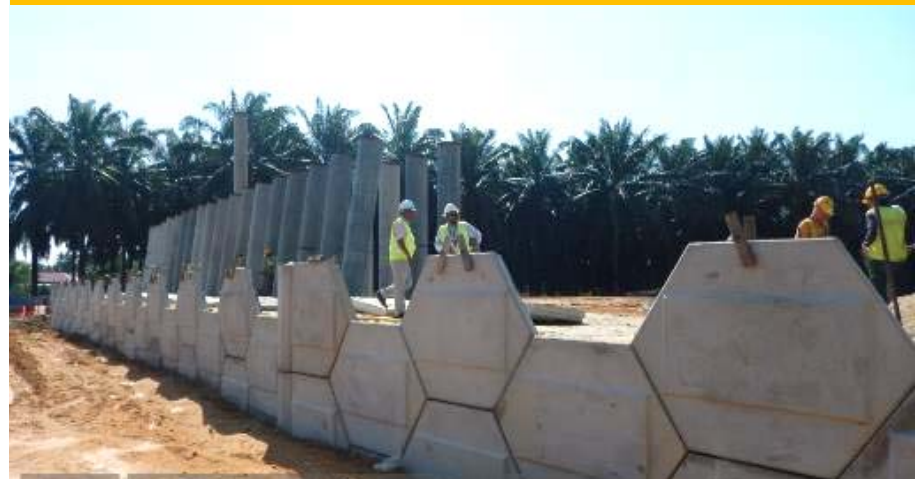
RS Wall Construction in Progress
