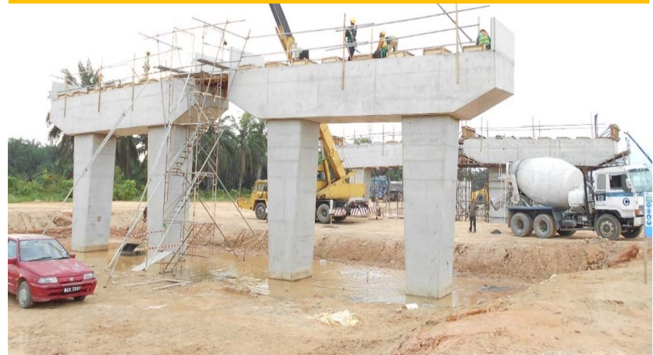
Concrete Casting Work for Bridge Plinth
