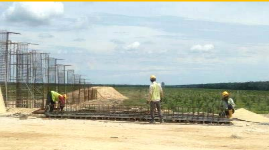
Construction of Precast Plank
