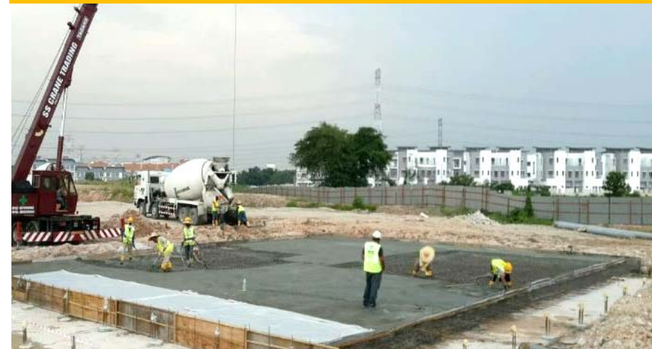
Concreting of Piled Embankment Slab
