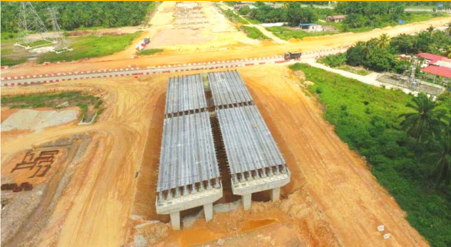
Construction of Precast Plank
