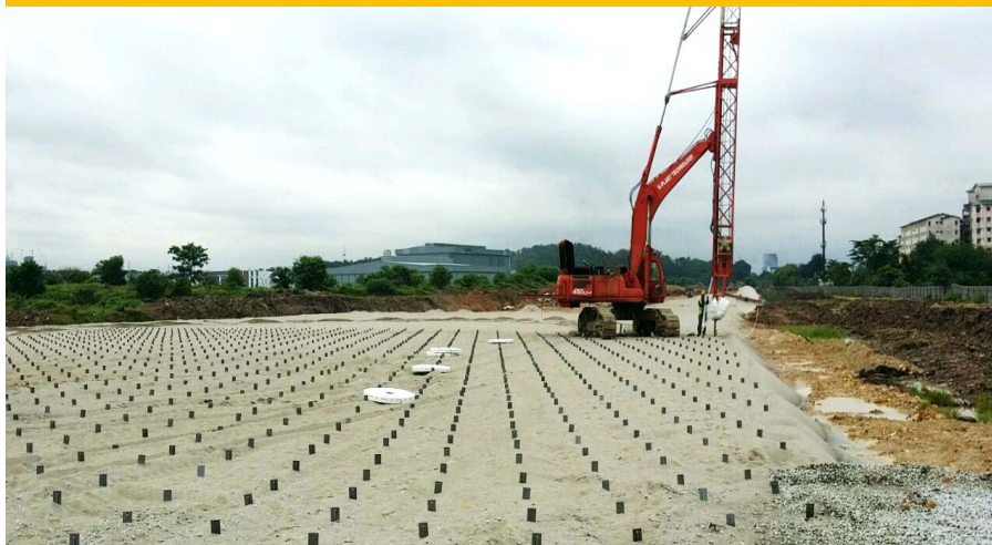
Installation of Prefabricated Vertical Drain
