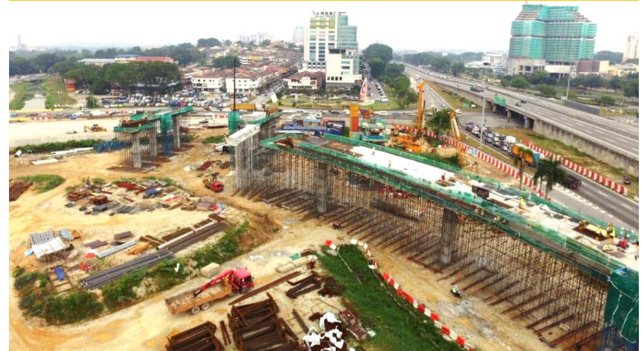
Installation of Rebar for Bottom Slab & Web of Multicellular Deck
