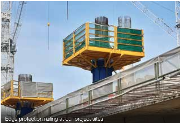
Edge protection railing at our project sites
