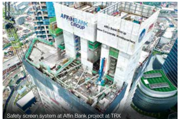
Safety screen system at Affin Bank project at TRX
