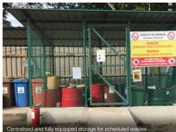
Centralised and fully equipped storage for scheduled wastes
