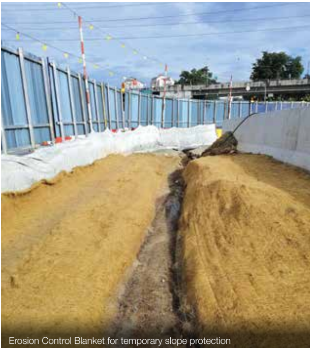
Erosion Control Blanket for temporary slope protection
