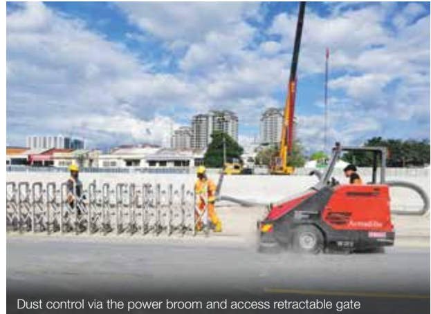
Dust control via the power broom and access retractable gate
