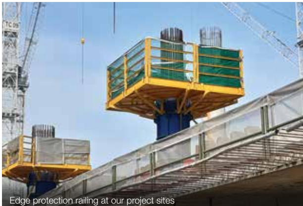
Edge protection railing at our project sites
