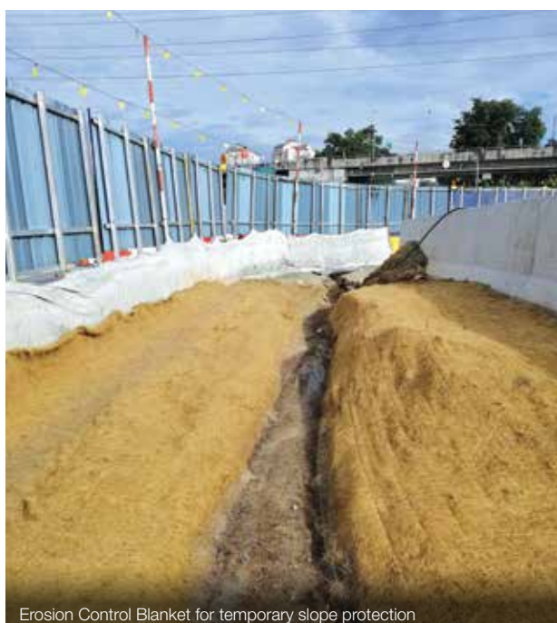
Erosion Control Blanket for temporary slope protection
