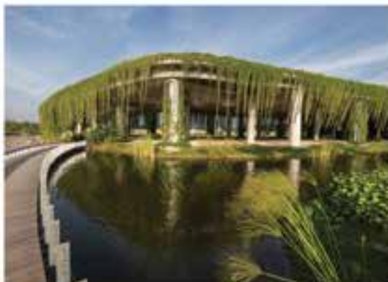
Elevated green roof with shade-providing curtain creepers
