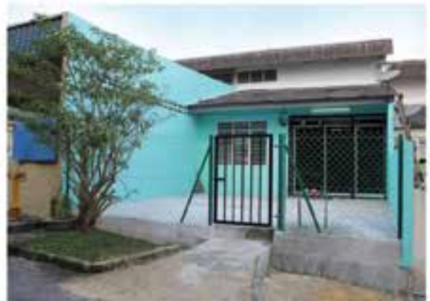
House condition after the Home Rehabilitation Programme
